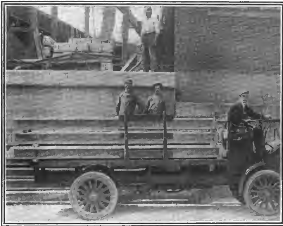
Universal 3-ton truck in the service of the Concrete Lumber Co., Detroit, Mich.
